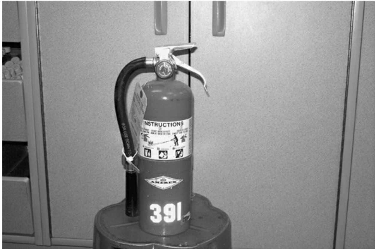
Figure 3-58 Portable extinguishers are marked to indicate what type of fire they should be used on.
