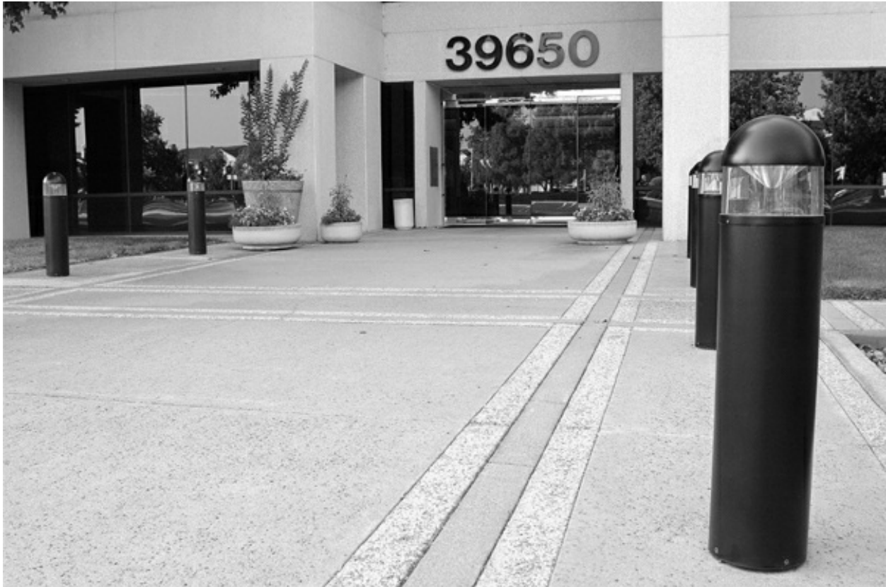
Figure 3-50 Sidewalks, lights, and landscaping can be used for protection.
